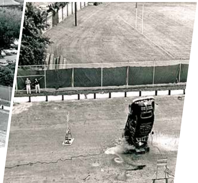
One of Ryan's testing methods involved dropping cars from cranes.
